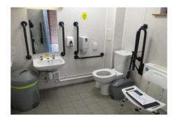
pan. The radiator to the side of the WC pan does obstruct transfer space slightly, having a depth of 140mm. The cubicle is fitted with an alarm system and pull cord.
