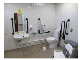
**Kettle Grove accessible WC and shower cubicle** door achieves a clear opening width of 940mm with a raised threshold of 20mm. The door is operated by a RADAR key available from reception. The cubicle size is 2950 x 1950mm. The cubicle achieves adequate wheelchair manoeuvring space to shower and WC positions. The level access shower and WC are left hand transfer. The WC, basin and shower have ergonomic lever style controls and contrasting grab rails. The cubicle is fitted with an alarm system.
